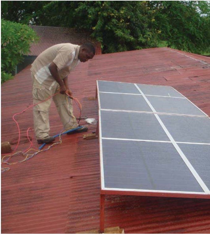
Installation of solar panels at Kilwa Masoko /Photo by Kicheko/
